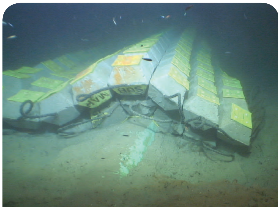
Articulated concrete mat protecting subsea pipeline. Photo: Submar.
