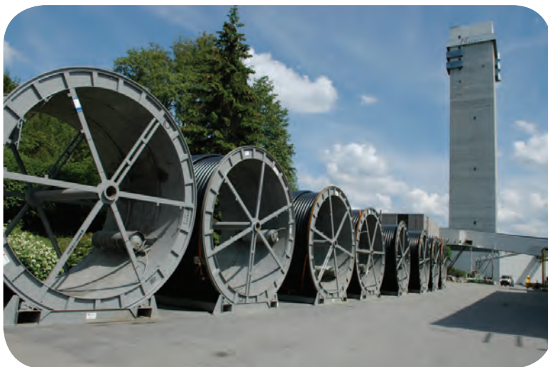
The Halden plant includes a 121m-high extrusion tower.
