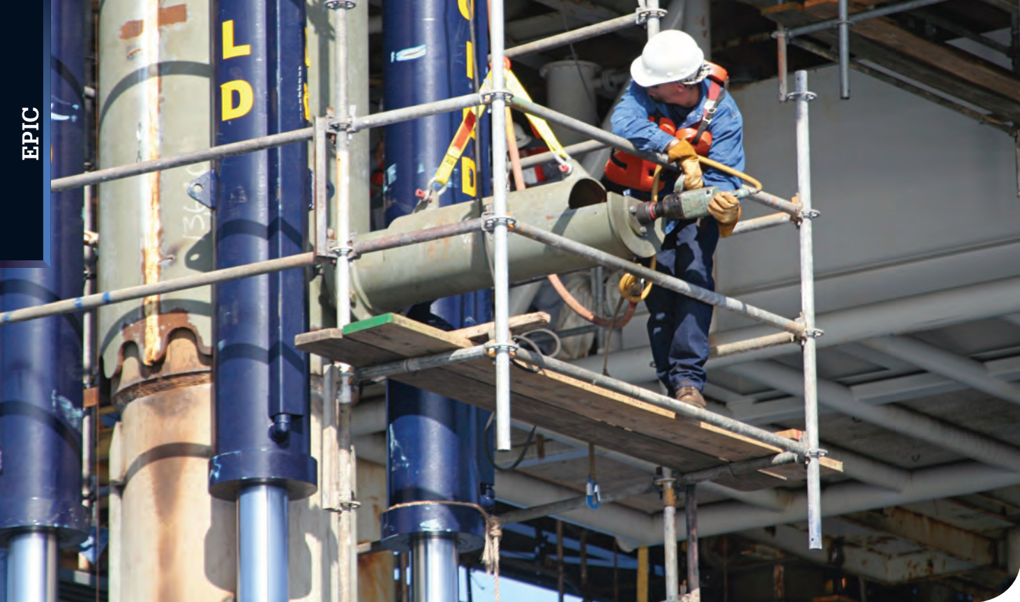
A worker installs a leg pin after jacking to raise the platform's deck.
