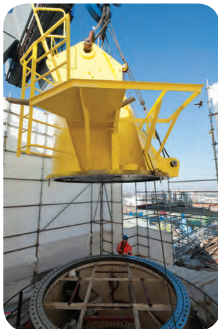
One of Gryphon Alpha 's three Hydralift hydraulic cranes being refitted.
