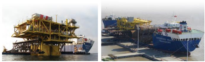
FIG. 4 & 5: TRANSPORT ARRANGEMENT AND SKID-OVER MATING WITH TOPSIDE SUPPORT FRAME
