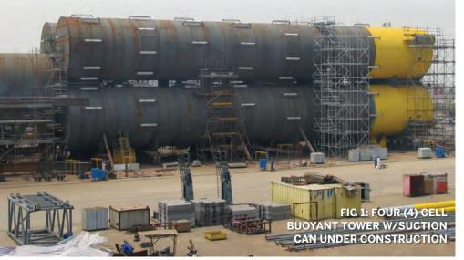
GMC Inc.'s Clyde Crochet discusses a self-installing tower, currently deployed off Peru, which offers a new substructure solution compared to conventional jackets/piles.
