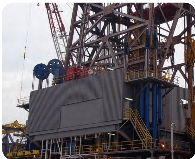
Tensioners in operation (colored in blue)
