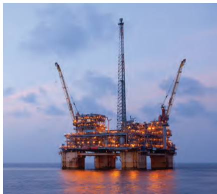
Located off New Orleans in the Gulf of Mexico, BP's Na Kika sits in 6300ft of water. Photo from BP.
