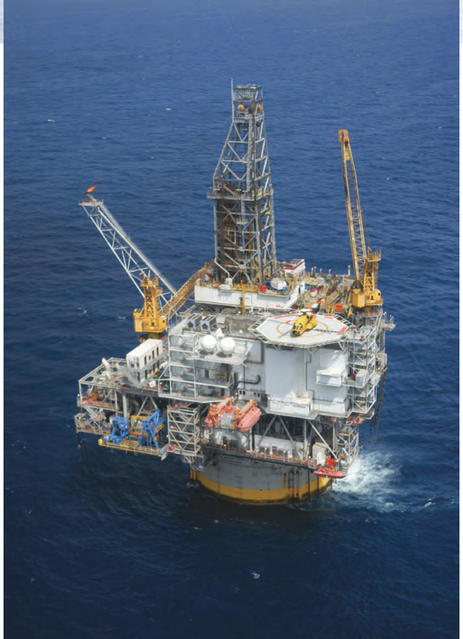
Located in the Gulf of Mexico in 4500ft of water, BP's Mad Dog platform can produce up to 80,000bod and 40 Mcf of natural gas per day. Photo from BP.
