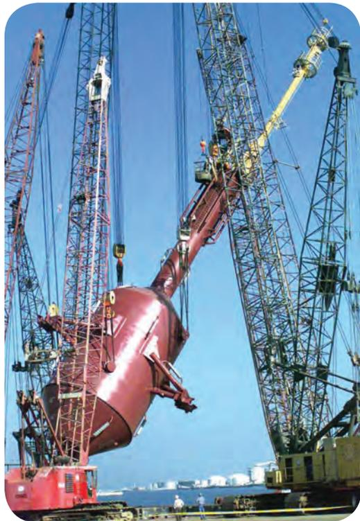
**Ocean Resource's production buoy concept under construction.**
