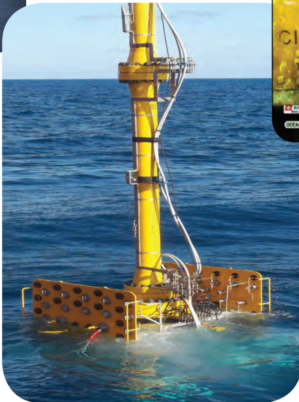
Deployment of the lower completion package.
