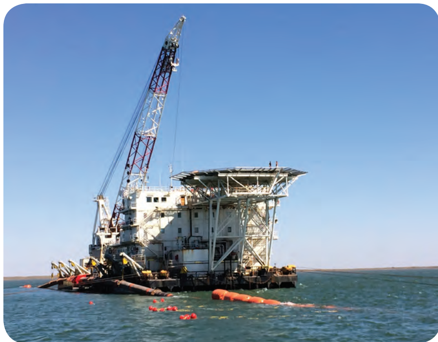
Allseas' Tog Mor flat-bottom, anchored barge used for pipelaying on Wheatstone.
