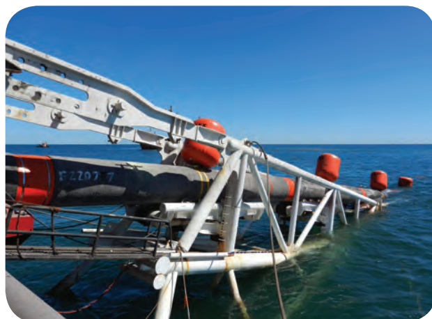
Inflatable buoyancy units during deployment on Wheatstone. Photo from Allseas.
