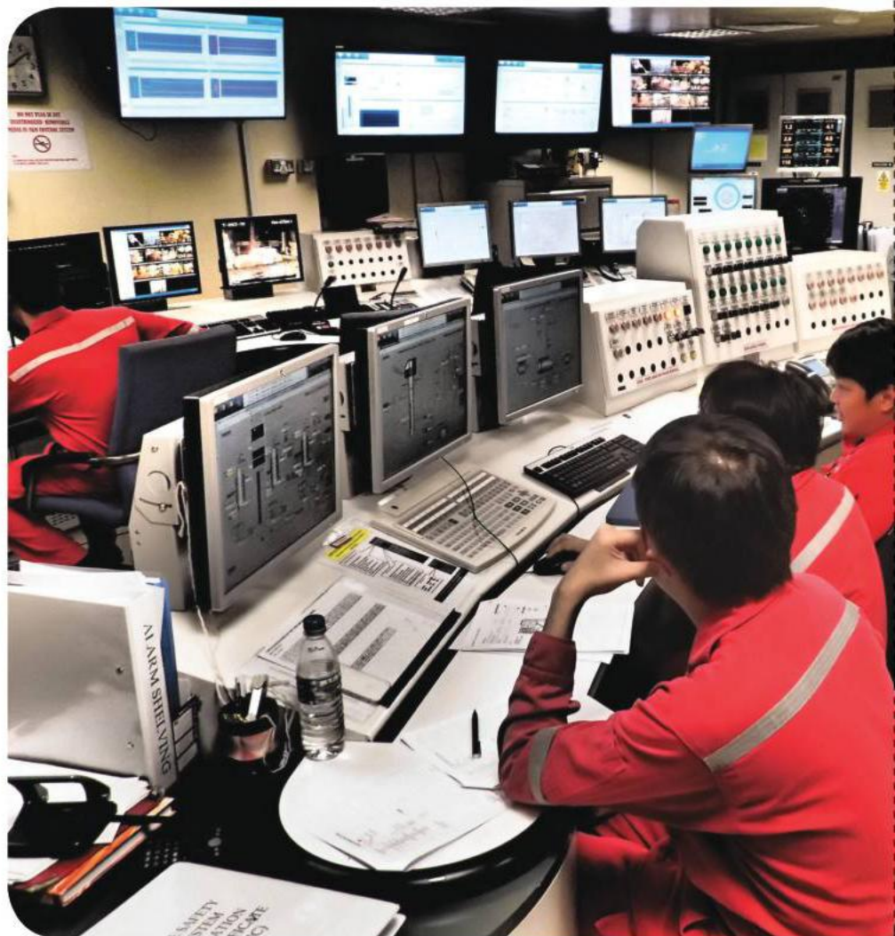
Engineers remotely monitor all aspects of oil production, and work across locations to make quick adjustments in Shell's Smart Fields control centers.
