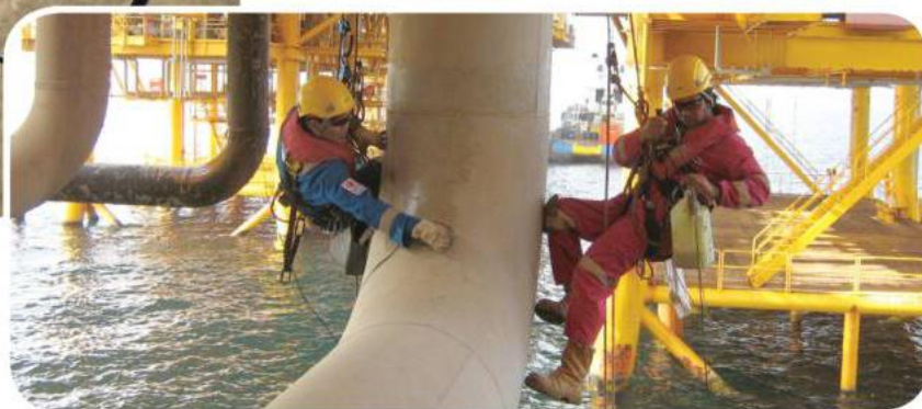
Workers perform inspection on an offshore installation. Photo from Oceaneering.
