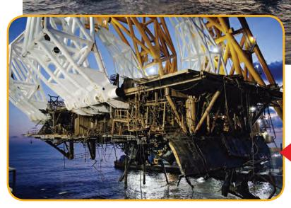
Peter Devine, of Versabar, sent in these photos of the company's heavy lift vessel, *VB 10000*, hard at work. The *VB 10000* decommissions a 2650-ton topside in the Gulf of Mexico. The twin gantries rise 260ft above the waterline. With a rated lift capacity of 7200-tons it is the largest lift vessel ever built in the United States.
