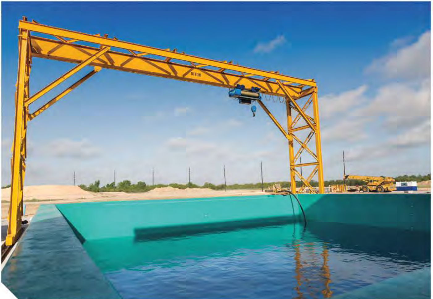
Seanic's new in-ground tank. Photos from Seanic.
