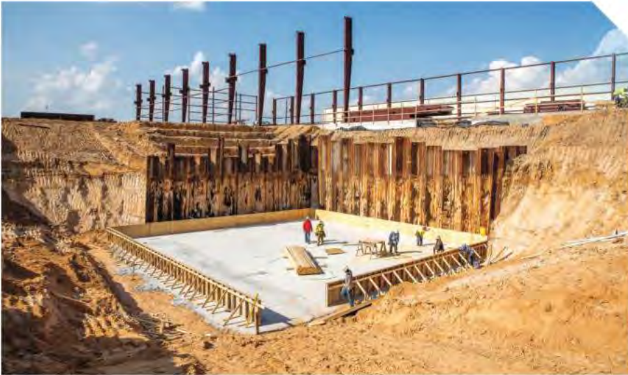
Construction on Seanic's tank at the deepwater hardware testing facility in 2015.
