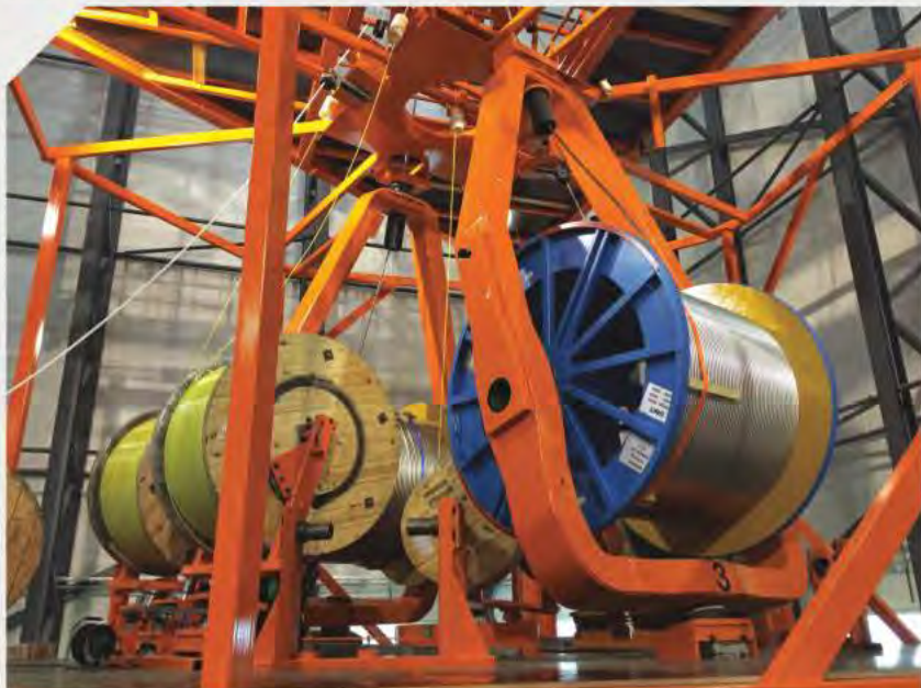
Unitech's umbilicals plant in Stord. Photos from Unitech.
