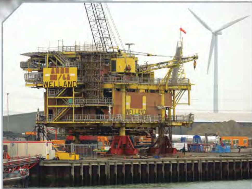
Since being removed in 2011, Perenco’s Welland platform topsides has been refurbished and re-installed offshore Cameroon as the Sananga 1 platform. Photo from Perenco.
