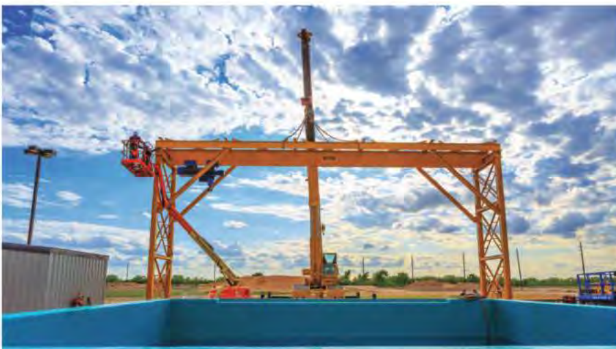
The gantry crane was installed in early April.
