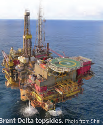
The Brent Delta topsides. Photo from Shell.
