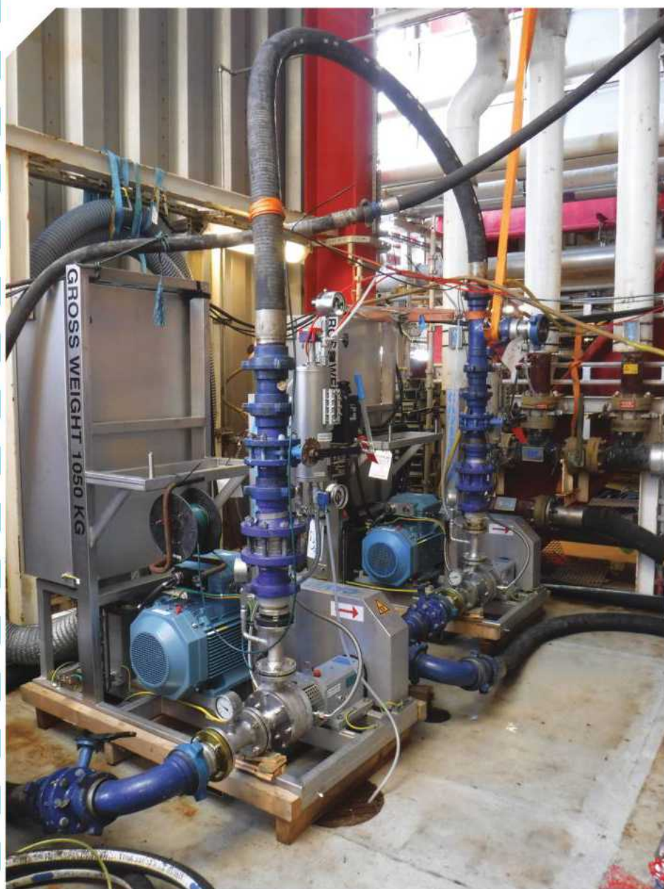
A cavitron mixer (a mixing unit for polymer and water). Photo from Statoil.
