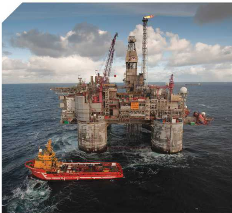
Statoil's Heidrun field. Photo from Statoil, by Øyvind Hagen.
