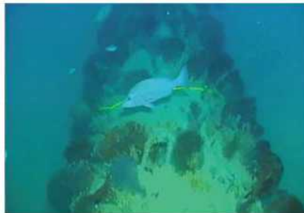
Operating pipelines provide habitat for marine life. Photos from Woodsid.
