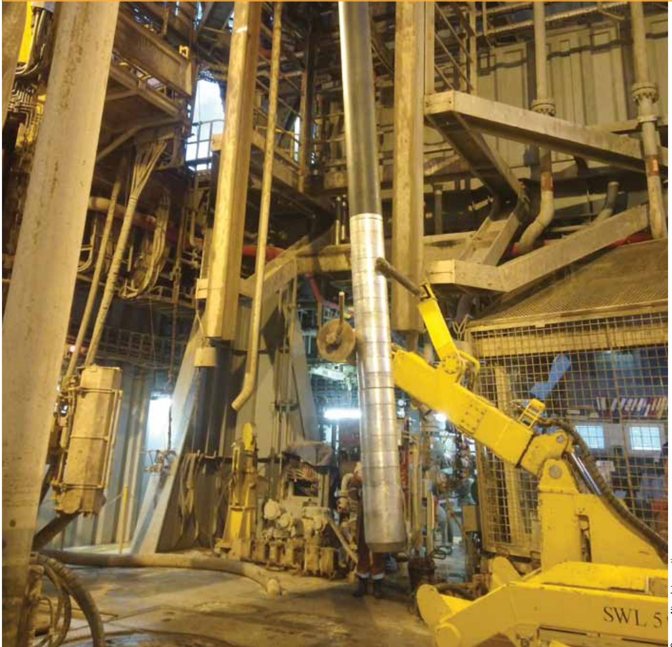
Source: Altus Intervention
