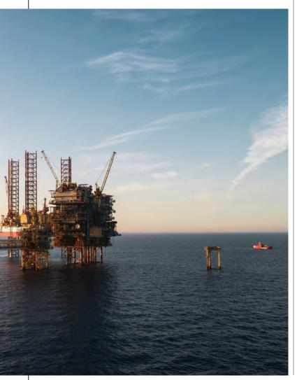
The removed topsides will be replaced by one new processing platform and one new accommodation platform. The four wellhead platforms and two riser platforms will have their jackets extended by 10-13 meters.
