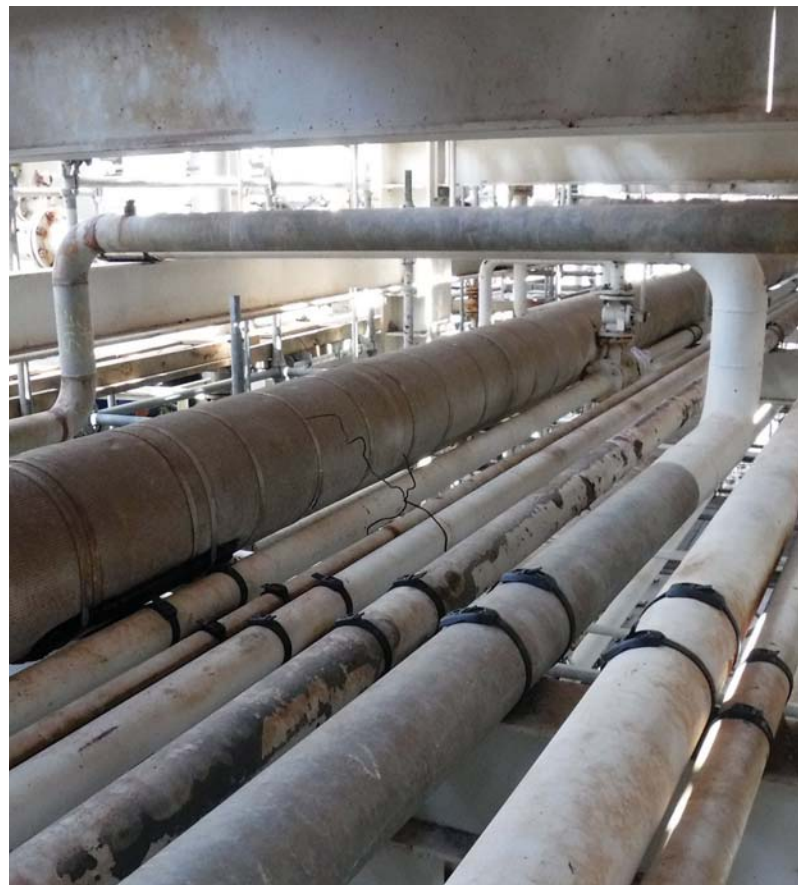
RedLineIPS SmartPads installed in a chemical plant's piping network at the Gulf Coast, providing long-term corrosion protection and improved airflow at critical support points.
